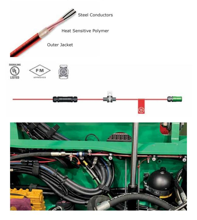
Large heavy-duty mining vehicles have large engine compartments. It is therefore important that the engine compartments are protected with additional suitable detection systems in addition to the linear heat detector which then provides the vehicle maximum fire protection.
